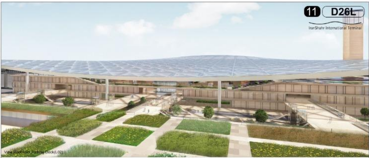
View Roof from Parking Deck(L02)
